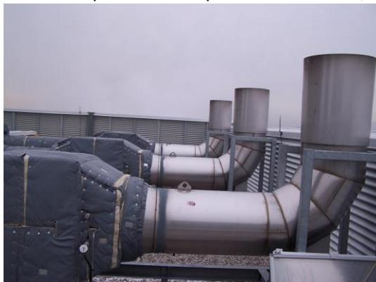
The Safety Power system met its design target of 90% reduction of NOx across a broad load range for each generator. These results make the system compliant with the current requirements of Ministry of Environment EBR 010-2463. In addition to dramatically reducing the NOx emissions, noise and visible particulates are also significantly reduced.
